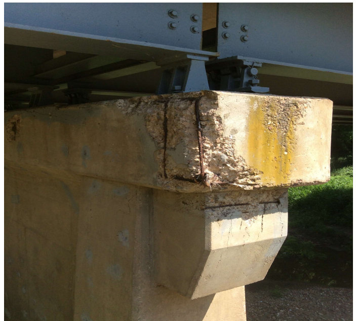
PHOTO 2 Description Bent 4 cap right has spalling with steel exposed.
