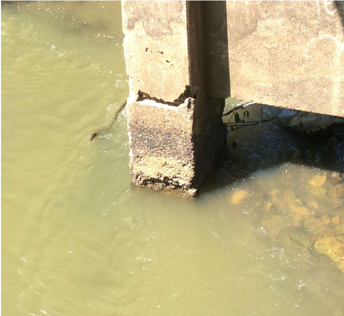
PHOTO 3 Description Bent 3 column 2 ahead side side large areas of spalling with steel exposed.
