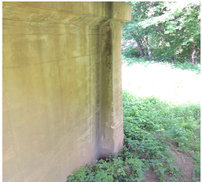
PHOTO 2 Description Bent 2 column 1 ahead side vertical cracking.
