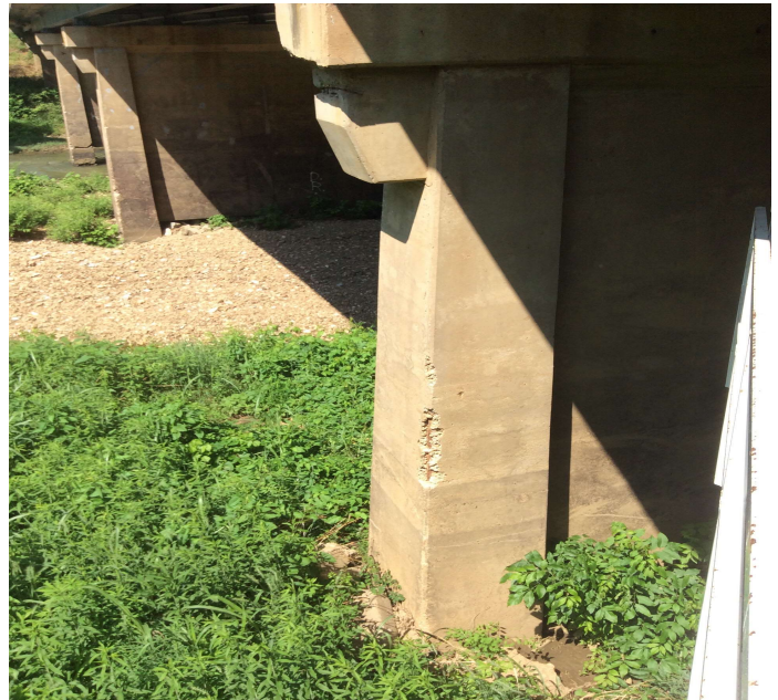
PHOTO 2 Description Bent 5 column 2 right side steel exposed.
