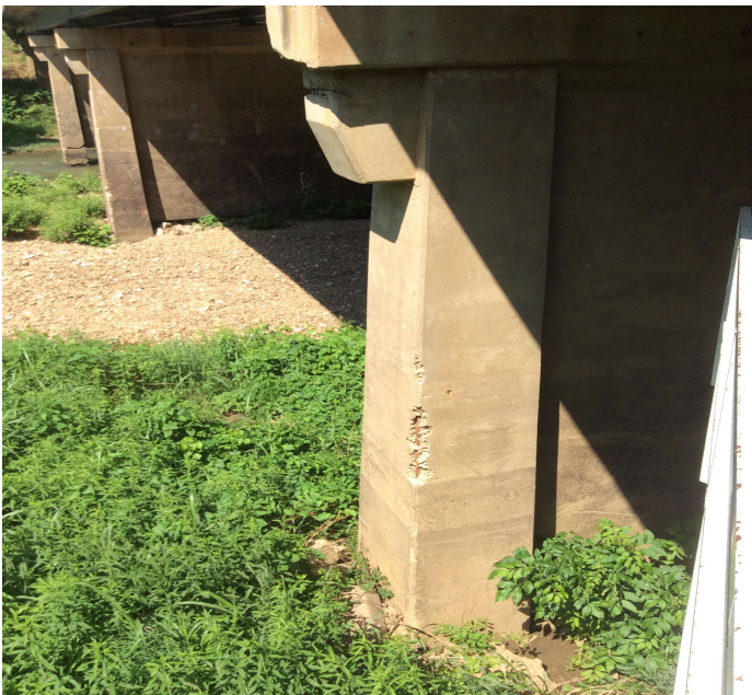
PHOTO 1 Description Bent 5 column 2 right side steel exposed.
