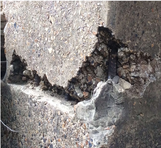
PHOTO 1 Description Bent 3 ahead side of right column 2 steel exposed.
