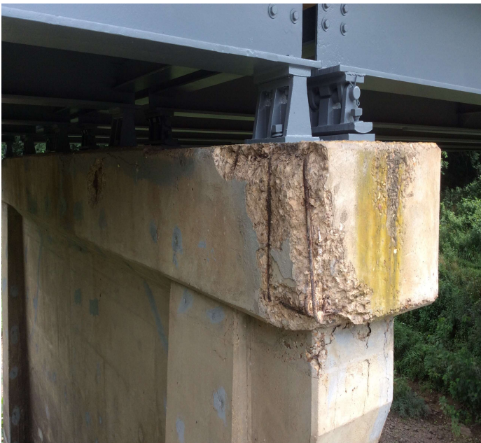
PHOTO 1 Description Exposed rebar to right end of bent 4.
