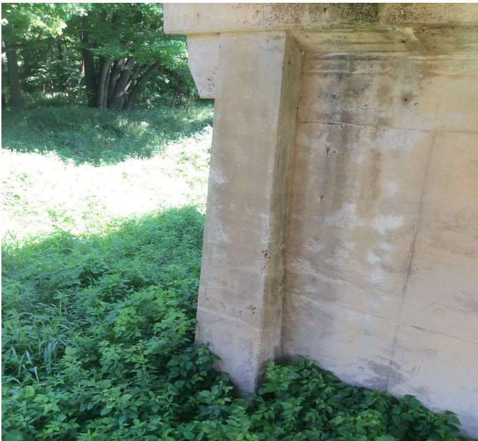
PHOTO 3 Description Bent 5 column 1 behind side sampling and cracking.
